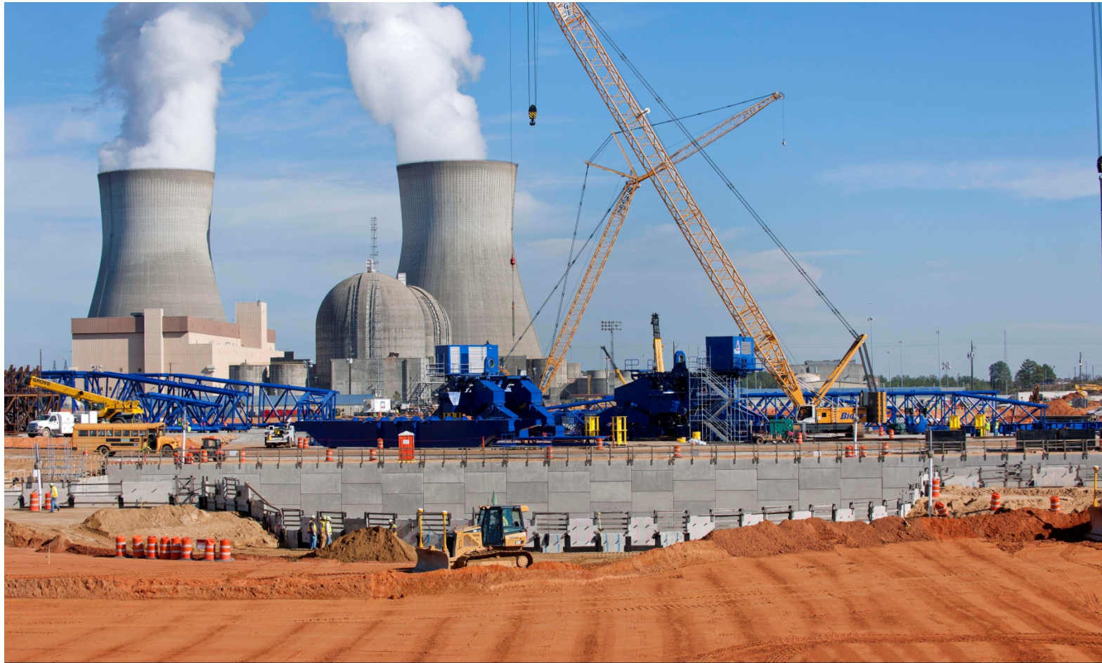
Vogtle Unit 4 nuclear island, heavy lift derrick assembly (blue), and Vogtle 1 and 2 operating units.
